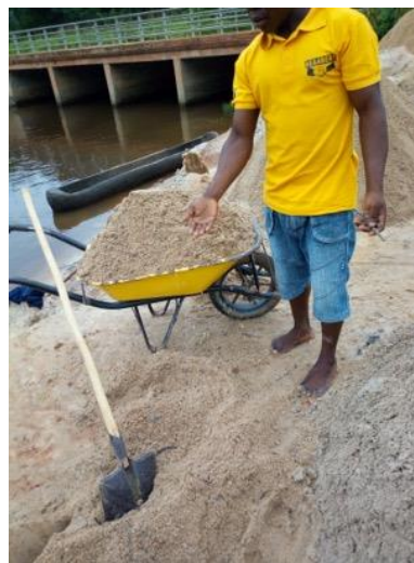
Figure 75: Workman at Longtimbi shows his working tools. In the background, boats are different than those in Yato
