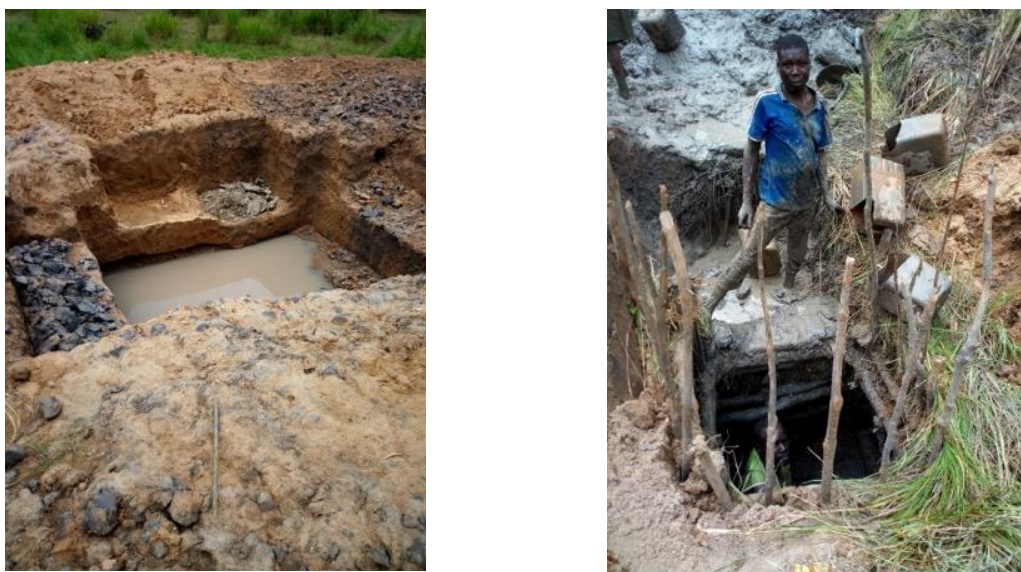
Figure 46: Environmental and community safe issues: excavation holes in sapphire mine site, Banyo
