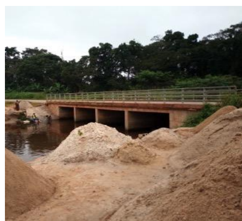
Figure 62: Paved access to sand loading site at for 4 wheel drive and motorcycles, Long-timbi
