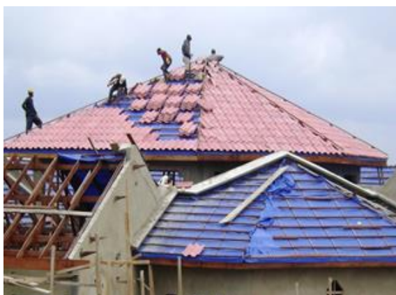
Figure 82: Micro-concrete roof tile used for roofing (Photo credit: MIPROMALO, 2017)
