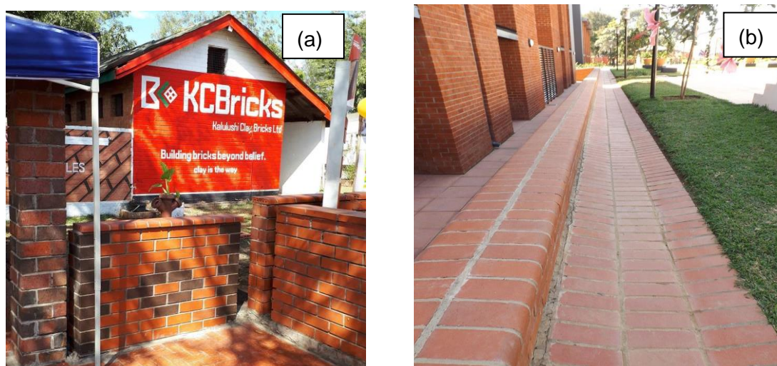
Fig. 21: Kalulushi Burnt Clay Bricks. Note bricks used for fencing wall and floor (a) and for and in drainage paving (b).
